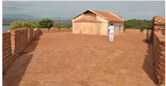
Flooring and Battlement : After Restoration
