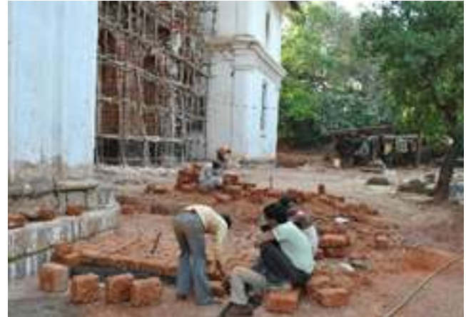
Plinth Protection : Before Restoration
