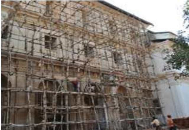
Northern Central Façade : After Plaster
