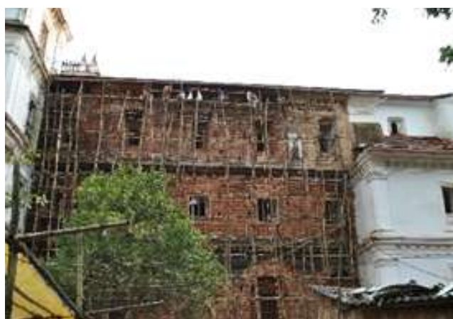
Northern Central Façade : Before Plaster
