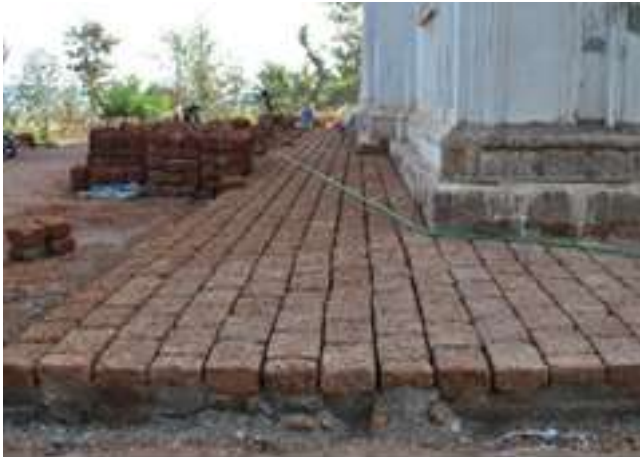
Plinth Protection : After Restoration
