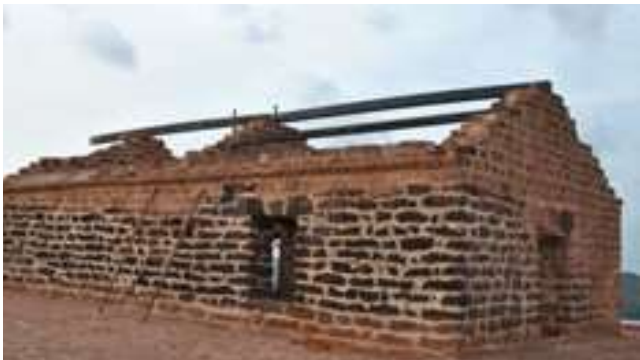
Restoration of the Central Chamber
