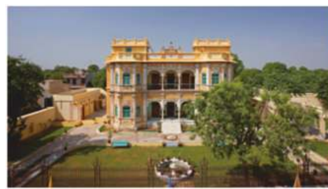
KoolwalKothi :Before Restoration
