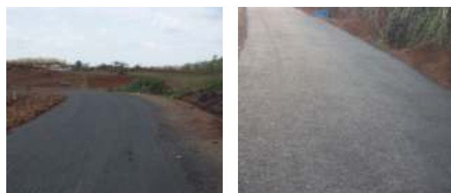
Figure 6 Final View of Rural Road by Cold Mix Technology
