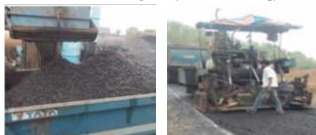
Figure 5 Laying of Green Roads by Cold Mix Technology
