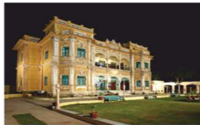
KoolwalKothi : After Restoration
